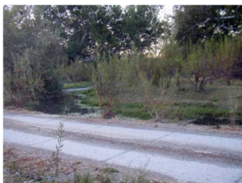
Photo #1. Looking down river, gravel is level with the concrete ford roadway. The Mocho is dry (10/9/2005) above the road and there is a 16½-inch drop to the water flowing in from the left, where the Zone 7-South Bay Aqueduct supplies water to recharge Livermore's underground aquifer.
