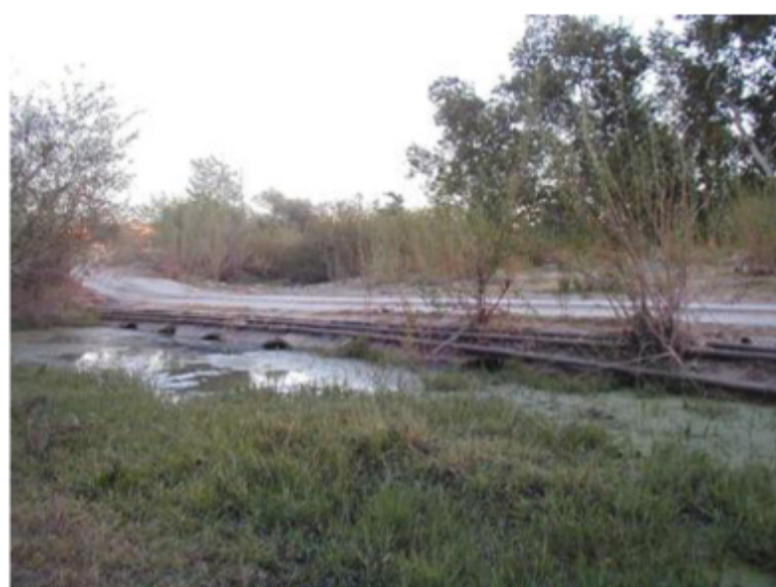
Photo #3. When the Mocho is flowing, it would pass over the ford in a very thin flow and drop to the stream below. In this photo the drop is 16½-inches. If the gravel were removed and kept removed from the upstream area above the pipes then there might not be a barrier to fish passage. Alternatively, the ford could be redesigned so that the flow over it allowed fish to pass upstream. The ford would have to be V shaped rather than flat.
